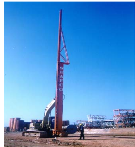
PVD equipment in operation
