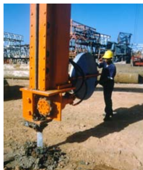
Close-up view of PVD installation
