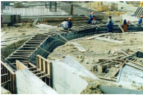
Guide wall construction.
