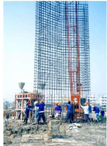
Installing a 24m-long reinforcement cage for a diaphragm wall panel.
