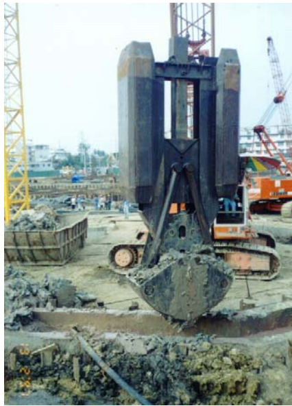
Diaphragm wall panel excavation.
