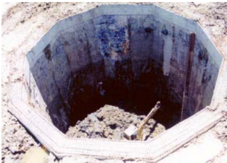
Excavation in progress.
