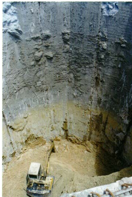
Excavation at depth about 20.0m below the ground.
