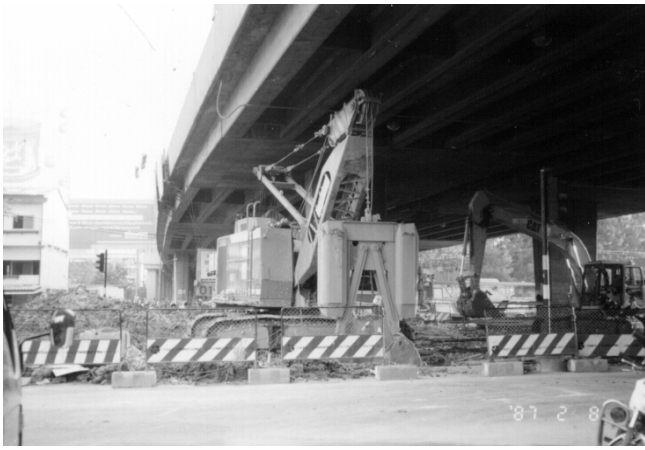
Figure 7 Specially designed baby-grab with short-boom for limited low-headroom area
