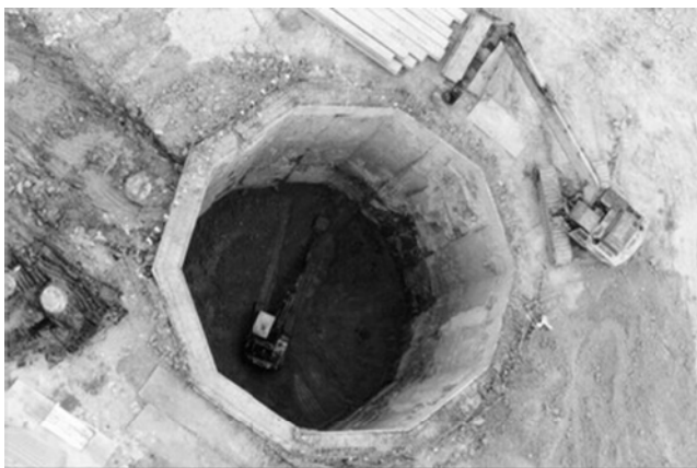
Figure 8 Deep circular shaft constructed by diaphragm wall
