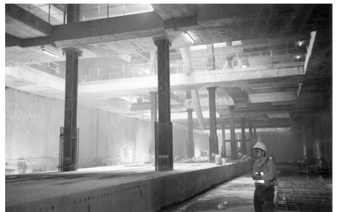
Figure 10 View of subway station construction with application of top-down method
