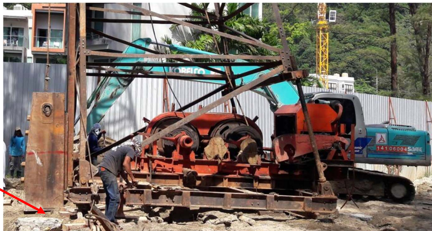
Fig. 8 Drop hammer for re-striking of bored pile
